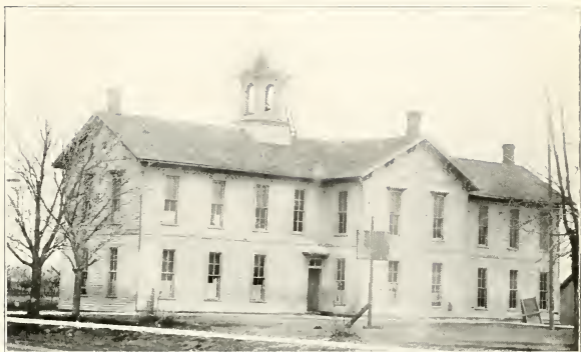
OLD PUBLIC SCHOOL BUILDING, JUNIATA
